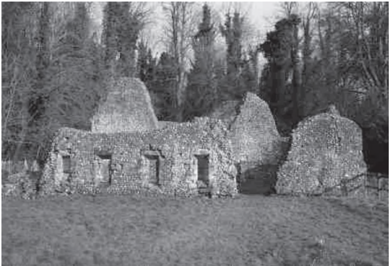
The remains of the house at Warnford that Adam de Port started to build in 1210 built of flints set in grout-work, 80 feet by 54 feet, with walls four feet thick. (photograph by Anthony St.John ©2005)
